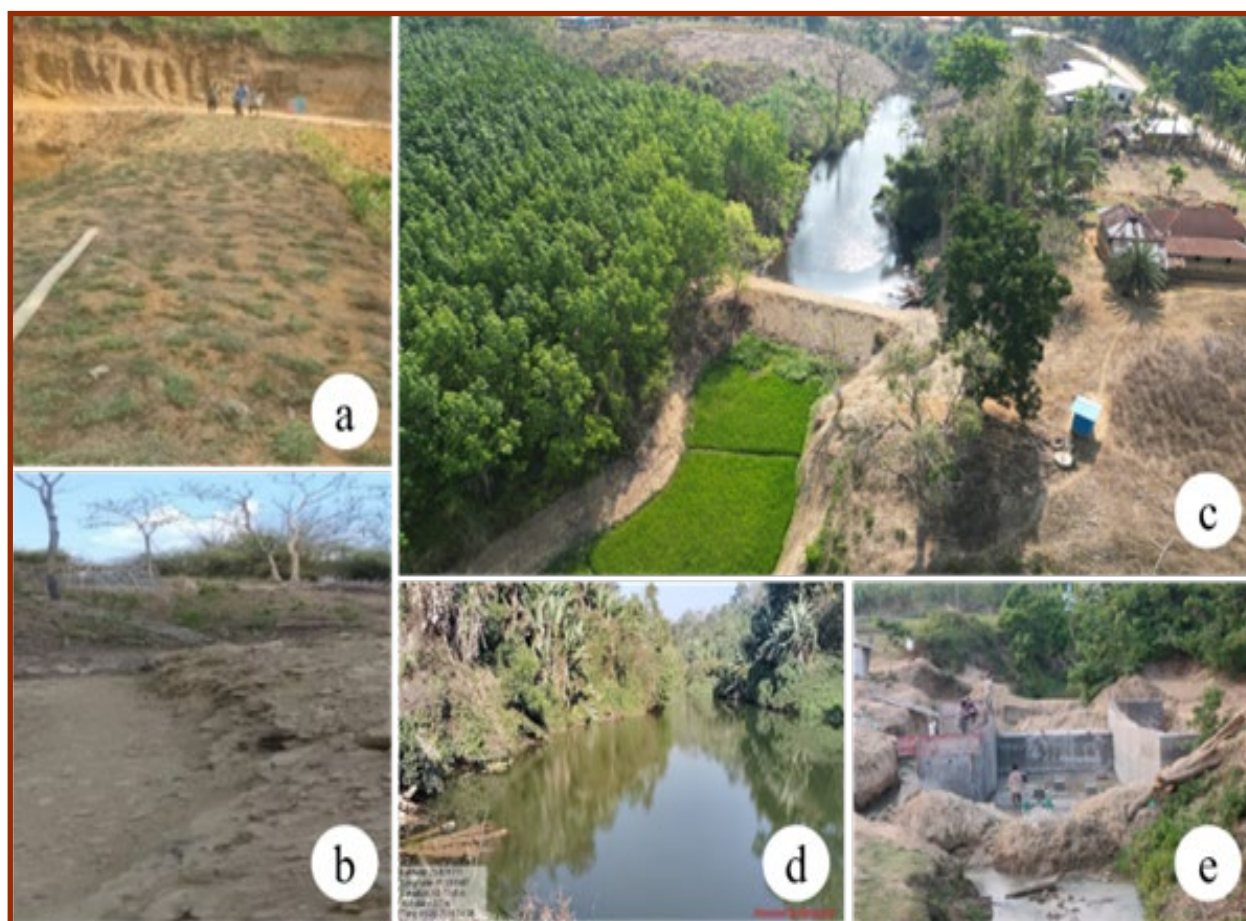
Figure 5: a-b) Model-I check dam construction at Panbagan JFMC (Balanancherra Beat); c) Model-II Checkdam (2024-25) at Matimapara JFMC, Gandacherra; d) Model-II check dams at Kathiram Bari JFMC (West Tripura); e) a Model-III check dam at Magroom Beat, Bankul RMU, South Tripura.
