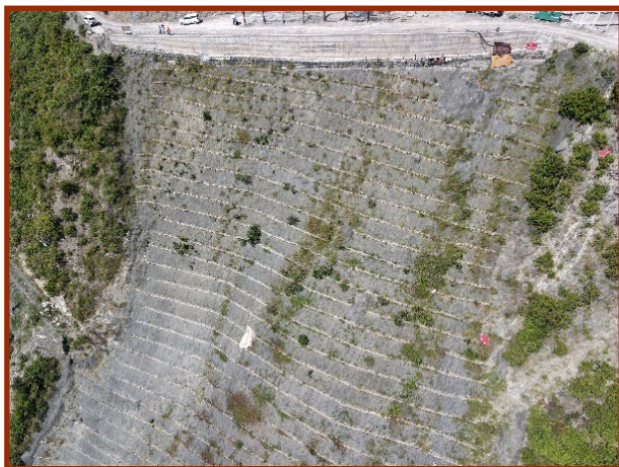
Crib work at Jawadi
